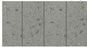
Integral color concrete sidewalk with sandblast finish and saw-cut joints.
