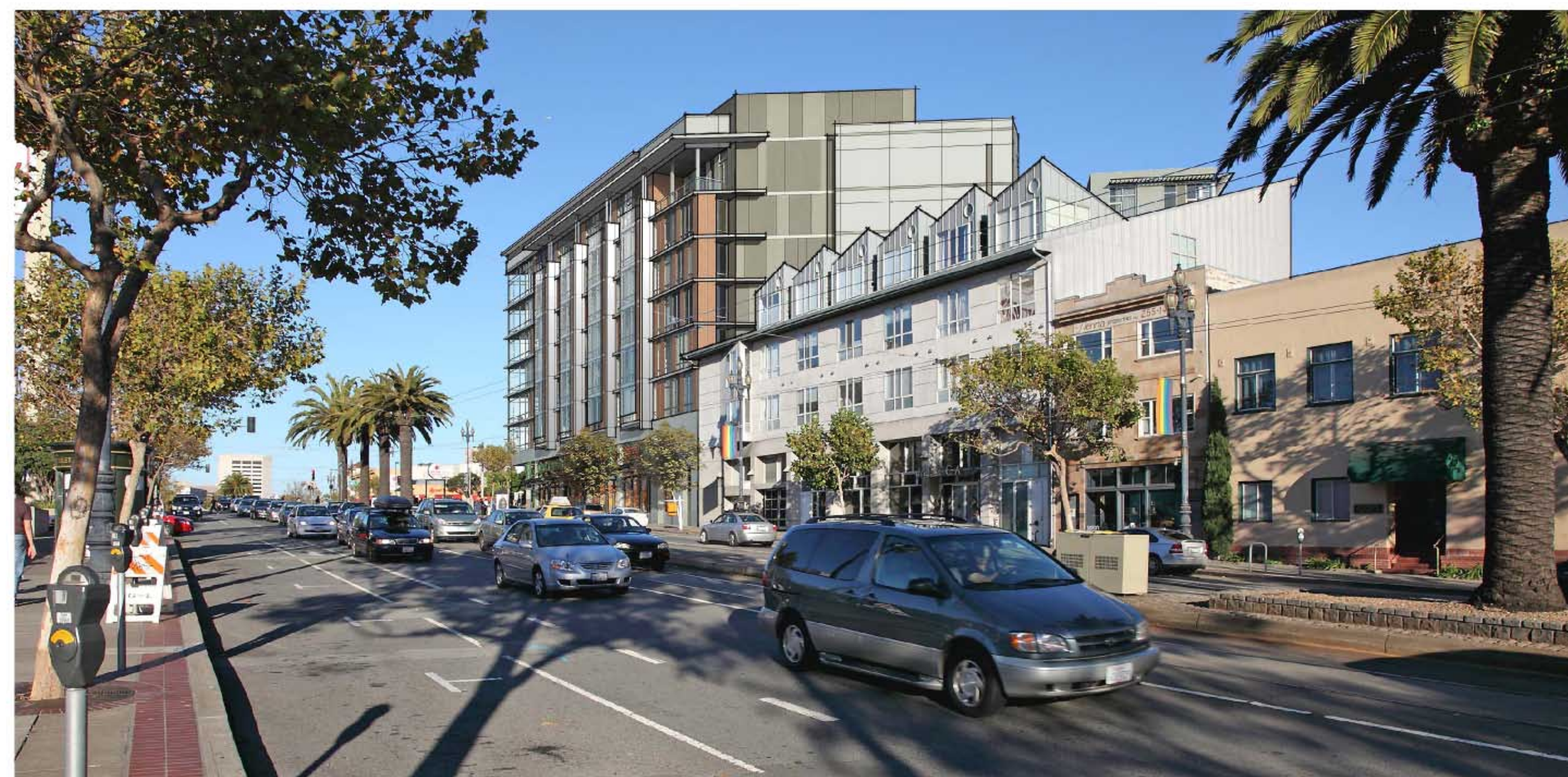
WEST FACADE VIEW
