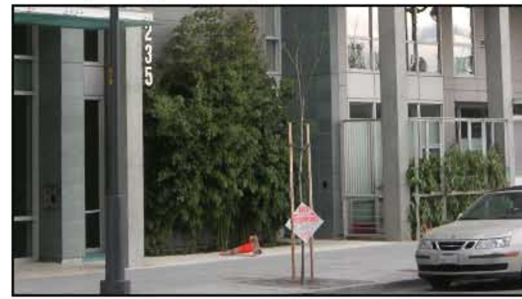
11 EXPOSED CONCRETE COLUMNS
