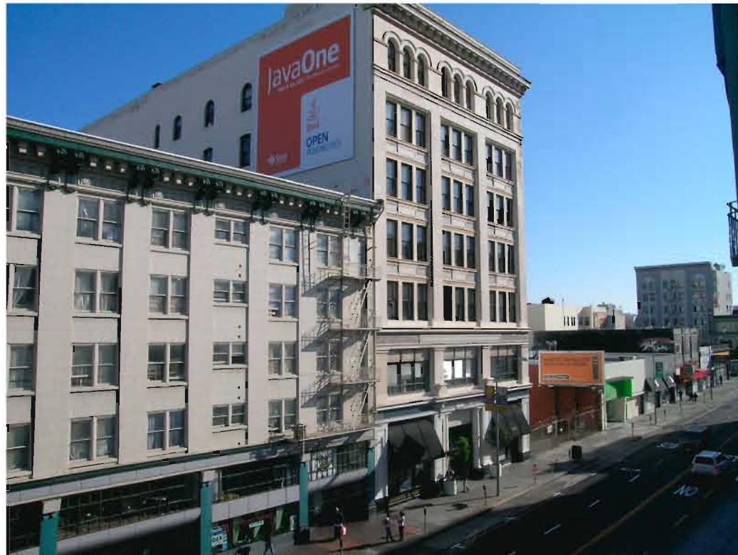
1 VIEW ACROSS MISSION STREET FROM 3RD FLOOR OF EXISTING BUILDING
