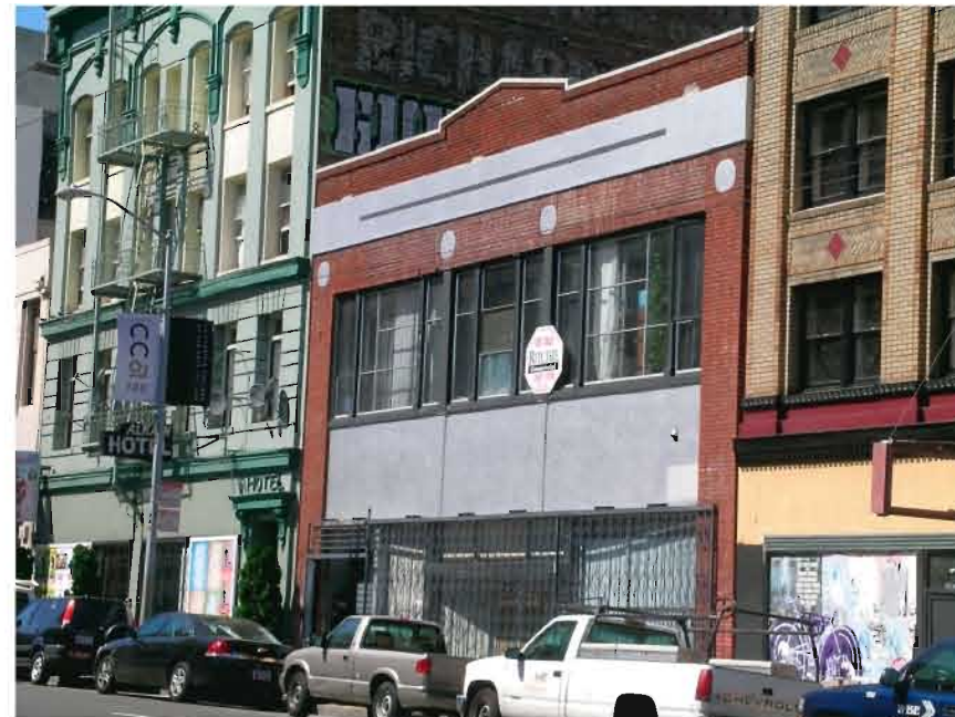
4 VIEW OF EXISTING BUILDING ACROSS MISSION STREET
