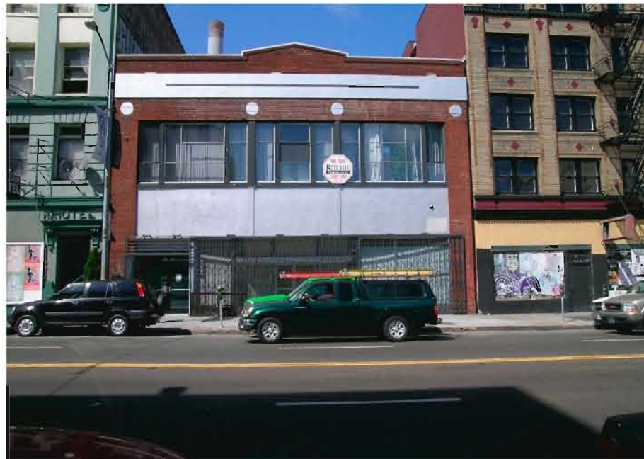
3 VIEW OF EXISTING BUILDING ACROSS MISSION STREET
