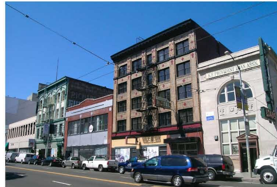
5 VIEW OF EXISTING BUILDING AND SURROUNDINGS ALONG MISSION STREET
