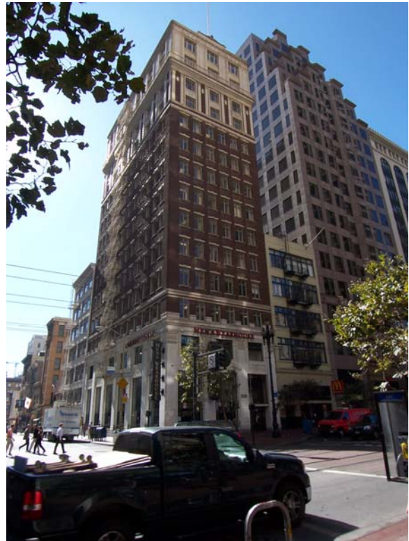
Figure 6. Santa Fe Building, 2007
