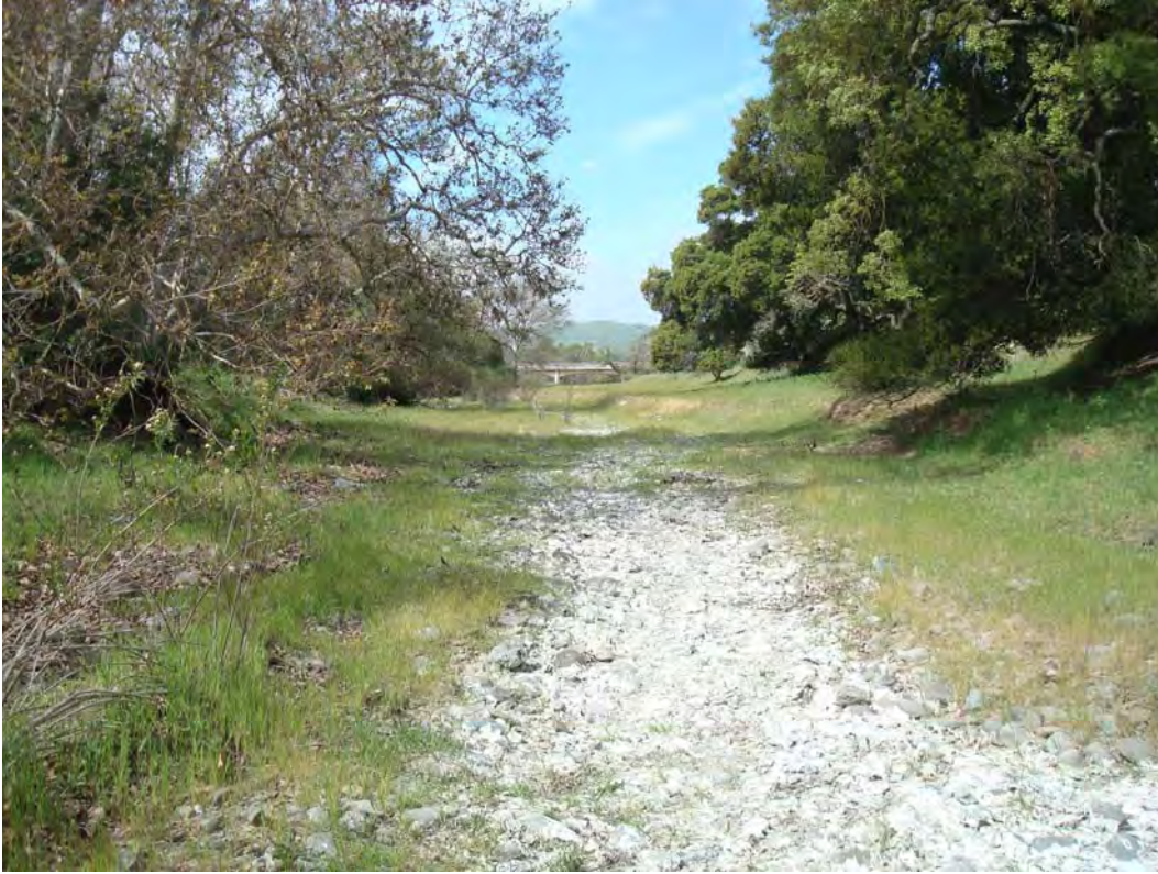
Photo 6: Looking west toward the bridge on Calaveras Road (IS-1).
