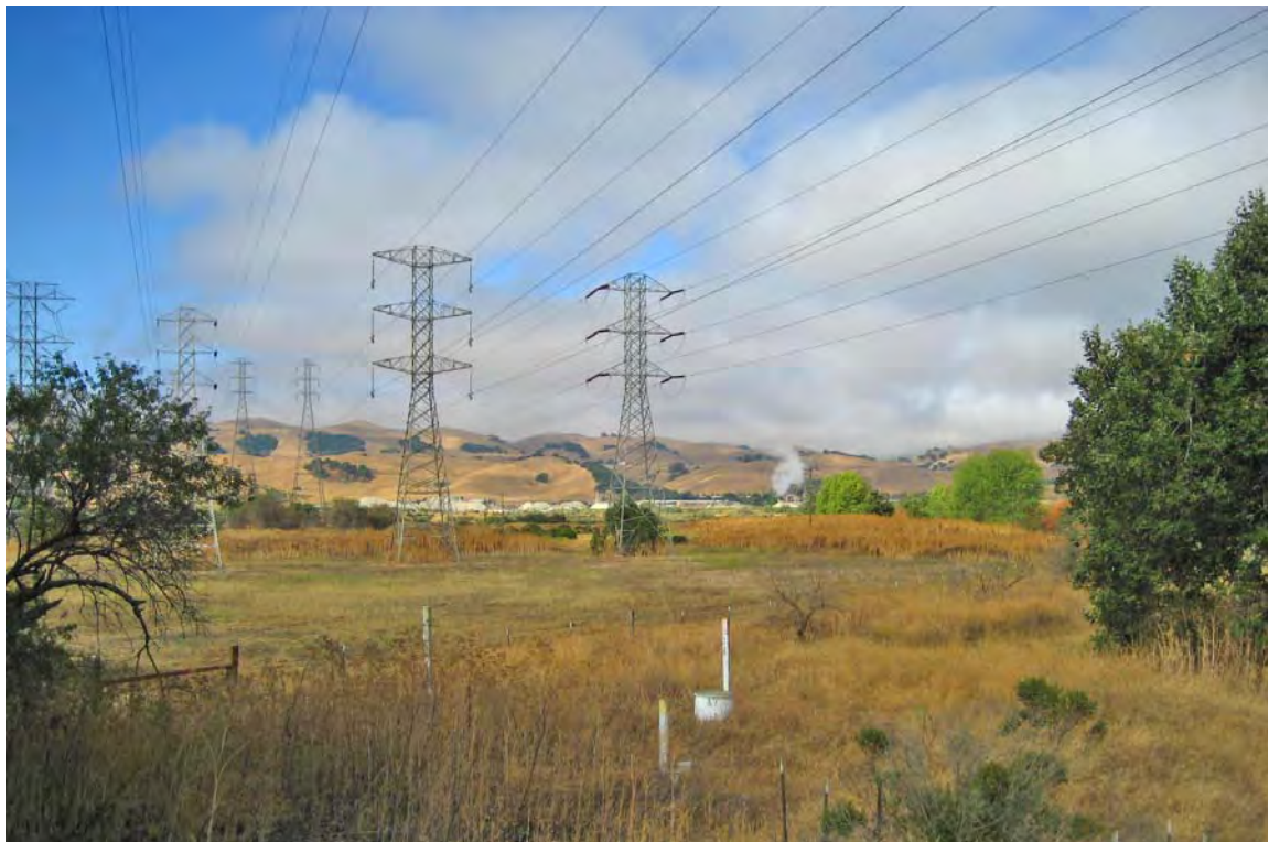
Photo 2 - View of Staging Area B looking southwest from Calaveras Road.
