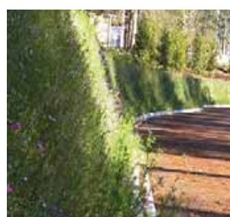
vegetated reinforced slope
