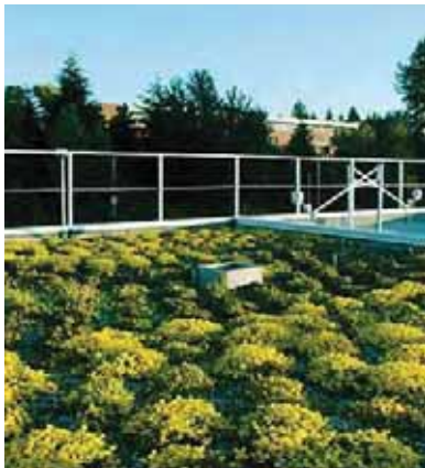
Green roofs can provide common open space.
