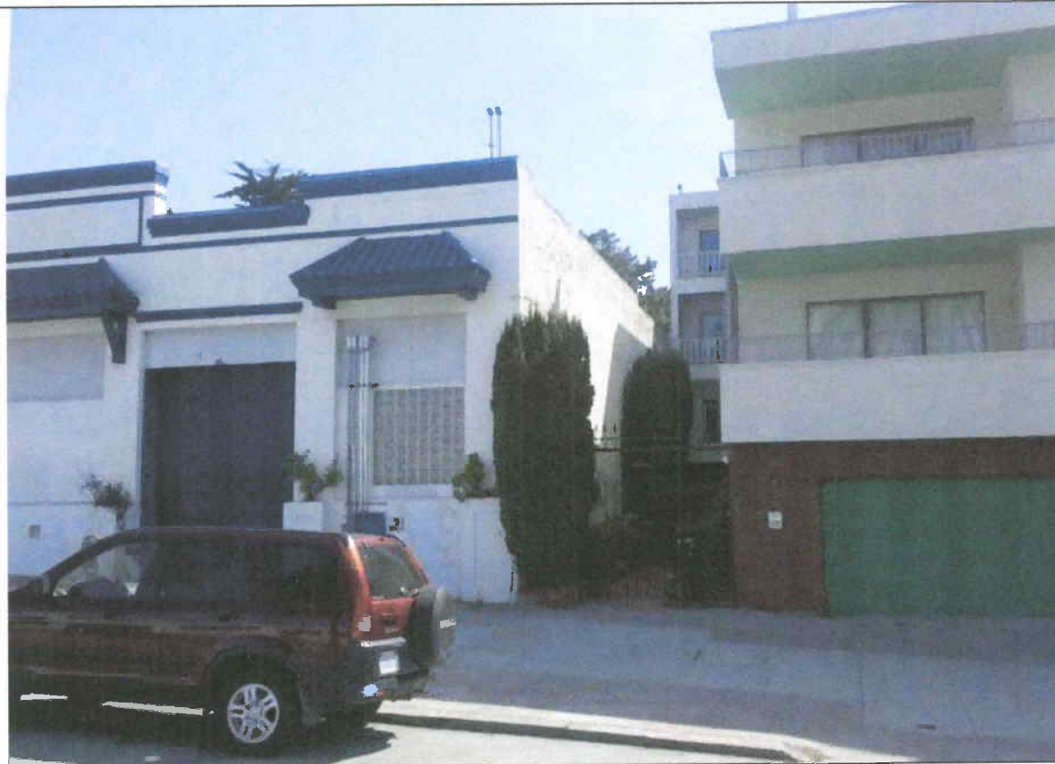
Front elevation of 23-35 Dolores and 55 Dolores Street. Note that the entryway gate for 55 Dolores is attached to the wall of 23-35 Dolores Street.
