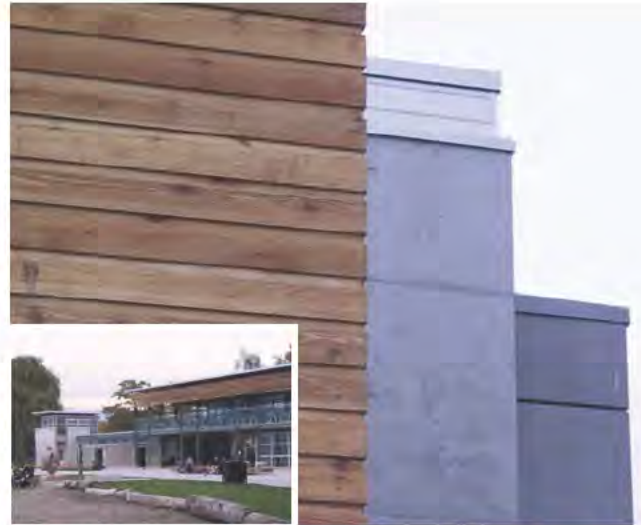
Combining a variety of good quality finishing material of wood, metal, and concrete create a rich and varied building facade.
