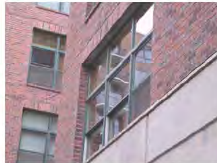
An good example of the use of brick with simply detailed windows relying on an ample recess as the major window detailing feature.
