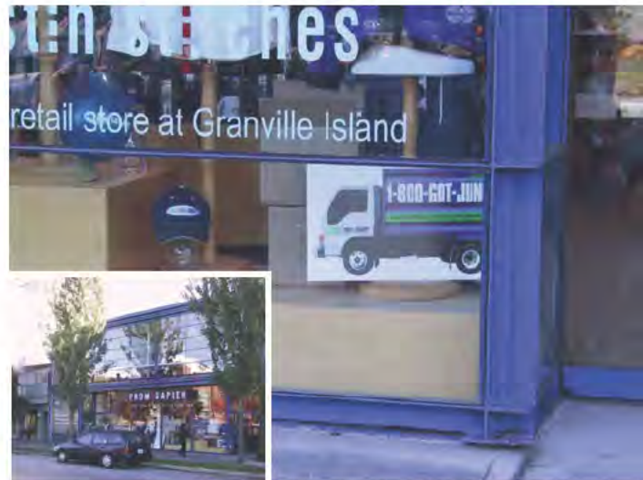
A well executed and honest application of fundamental and durable building materials of glass and steel.
