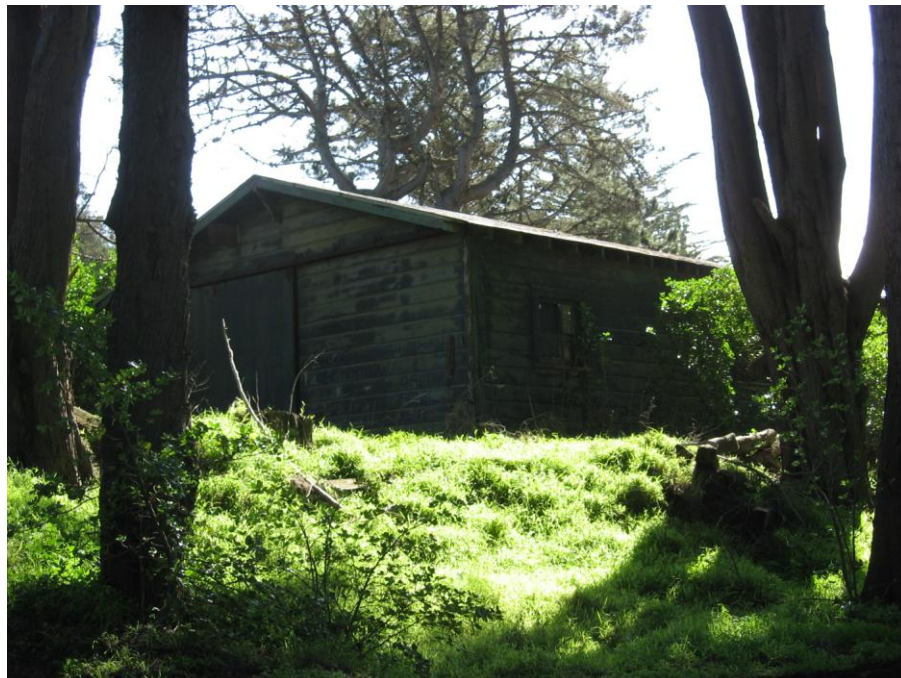
Photograph 11: Maintenance building, camera facing southeast, 3/4/2010
