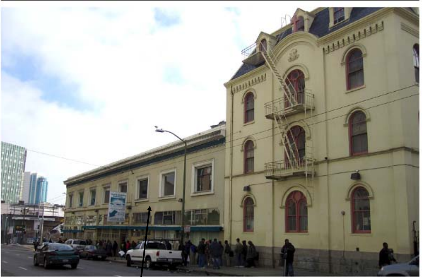
Golden Gate Avenue Looking East
