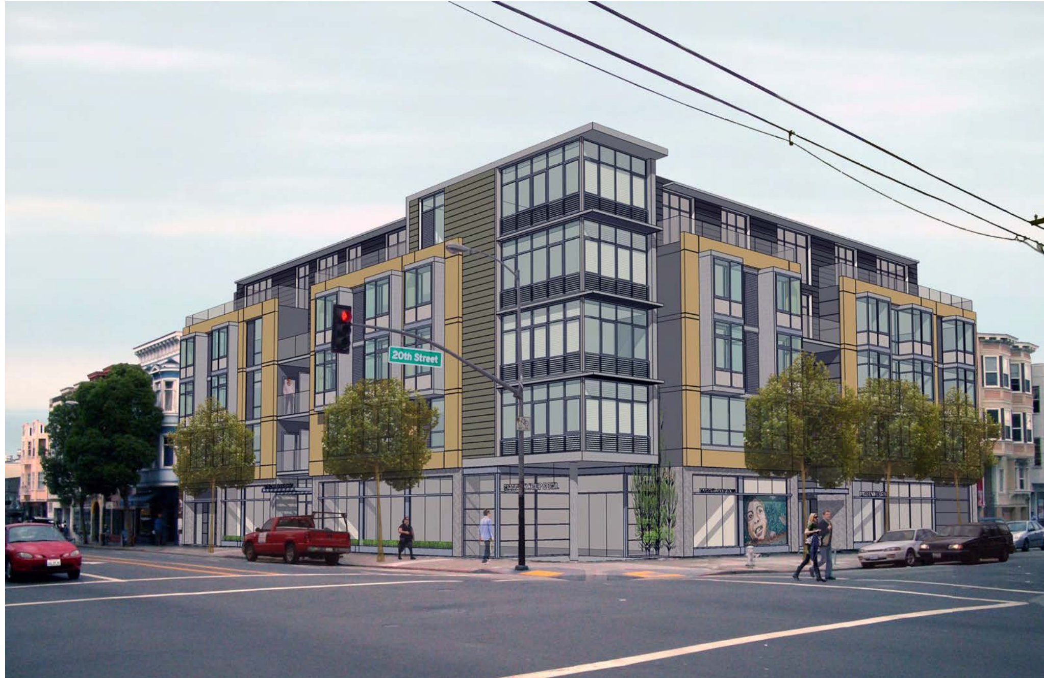
899 VALENCIA STREET NEW CONSTRUCTION MIXED-USE BUILDING
