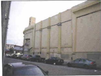
Theater To South Of Site
