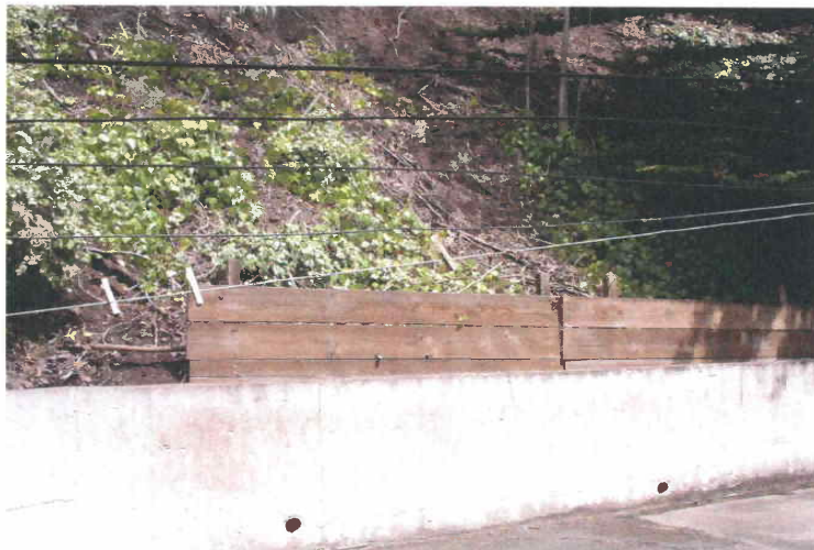
Picture #9: Retaining wall augmented to catch debris flow.
