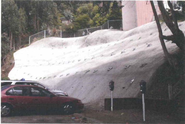
Picture #12: Concrete abutment with rock bolts at base of Kirkham Apartments
