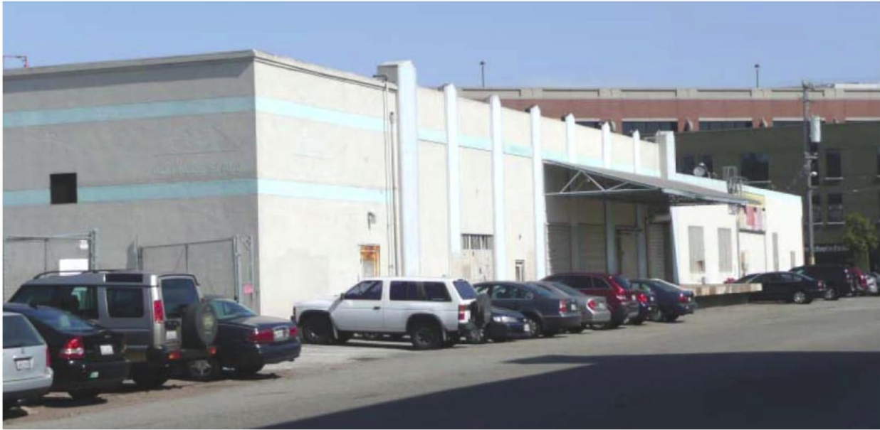
View Looking Northwest at Main Elevation
