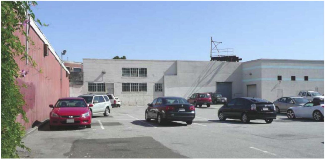
View Looking North toward South Elevation
