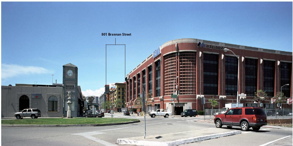
View with Proposed 801 Brannan Street Project
