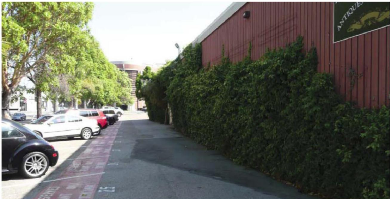
View Looking North along West Elevation 3-5 Henry Adams
