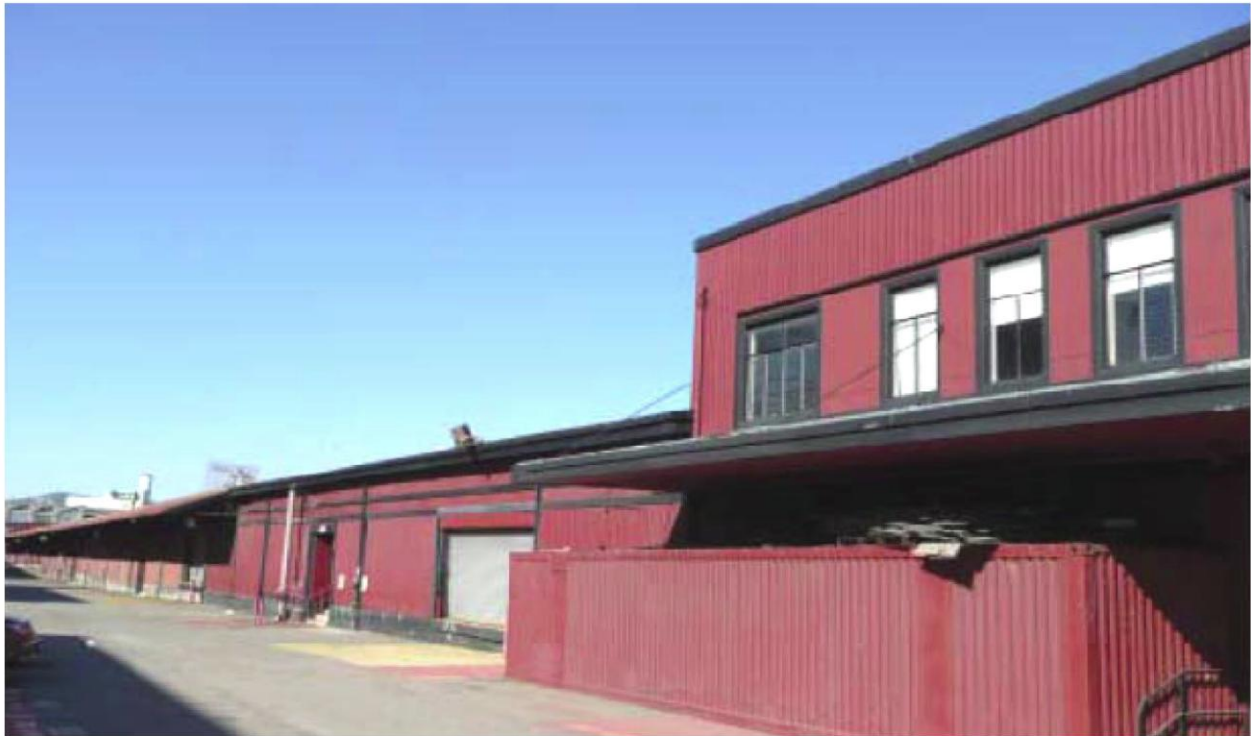
B. View Looking Northwest at South Concourse Elevation
