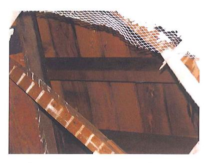
Photograph 16. Exposed Roof Framing and Sheathing
