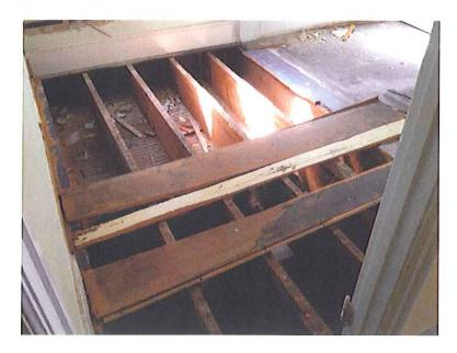
Photograph 14. Exposed Mezzanine Floor Framing
