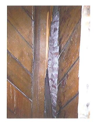
Photograph 6. South Wall Interior Showing Damaged Framing
