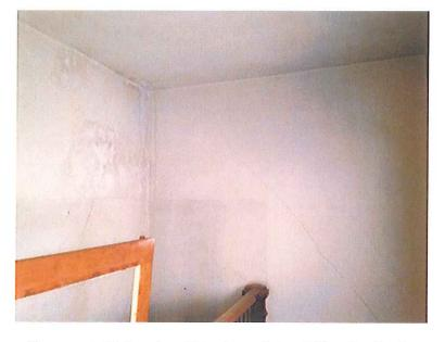
Photograph 11. Interior of Northeast Stairwell Showing Cracks
