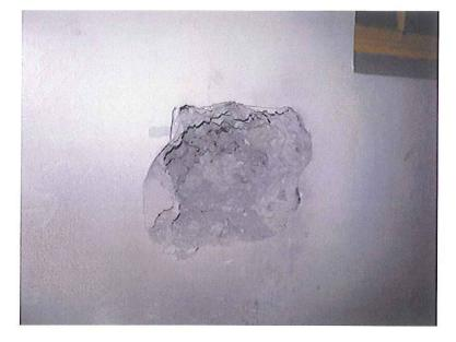
Photograph 13. Chipped South Wall in Basement Showing no Reinforcement in Concrete Wall
