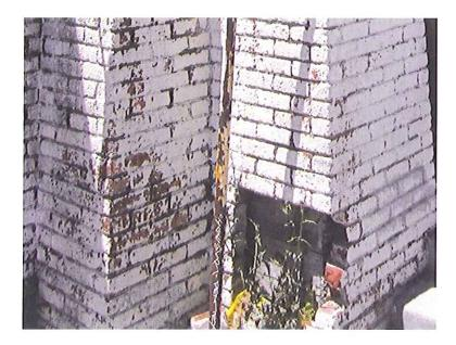
Photograph 2. Southeast Corner, Deteriorated Brick Veneer
