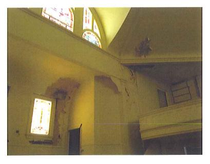
Photograph 9. Interior of Sanctuary Showing Water Damage
