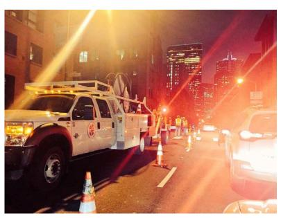
Crews laying fiber-optic (glass) cables under City streets. The signal from a mobile device, such a cell phone, communicates with the antenna on the pole. The signal would then travel from the antenna down through cables inside the pole to the radio relay units below. From there the signal would then travel through fiber-optic cables which run inside the pole and then underneath sidewalks and streets, through Pacific Gas & Electric conduit to the carrier's network hubs.
