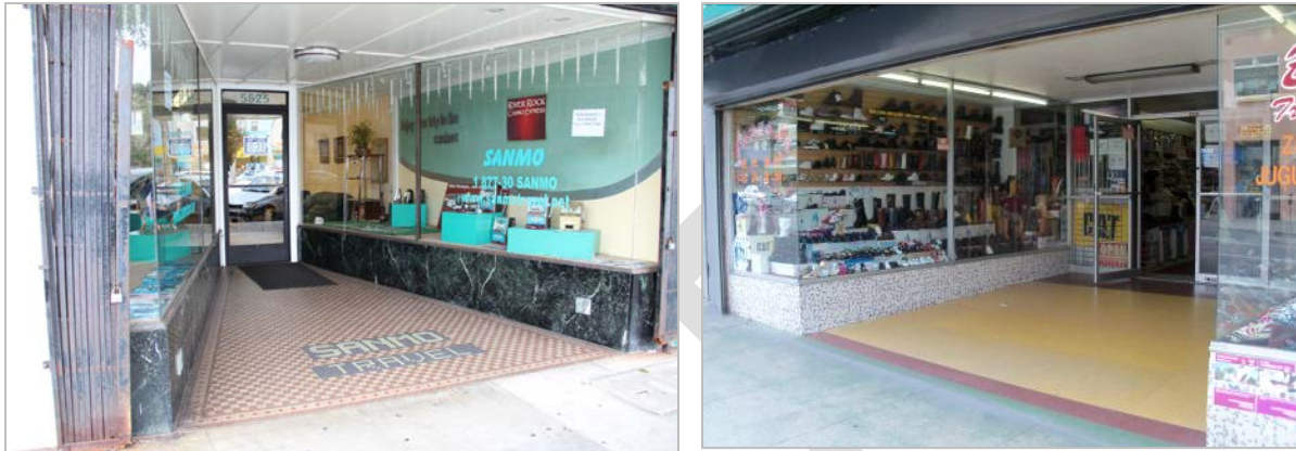
Left: Deeply recessed angled vestibule at 5521 Geary Boulevard. Center: Terrazzo paving on San Bruno Avenue. Right: A sample of terrazzo paving options. Source: “Mosaic & Terrazzo” (1931) and SF Planning
