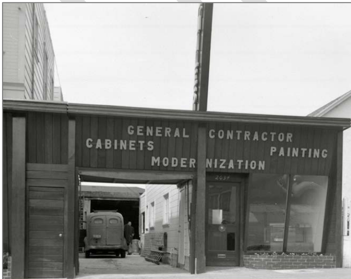
Left: 2034 Clement Street, unknown contractor's office. Extant, altered.
