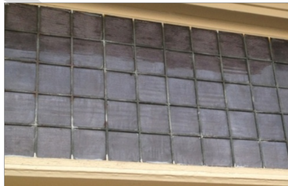
Below: Prismatic glass detail of 980 Valencia Street.
