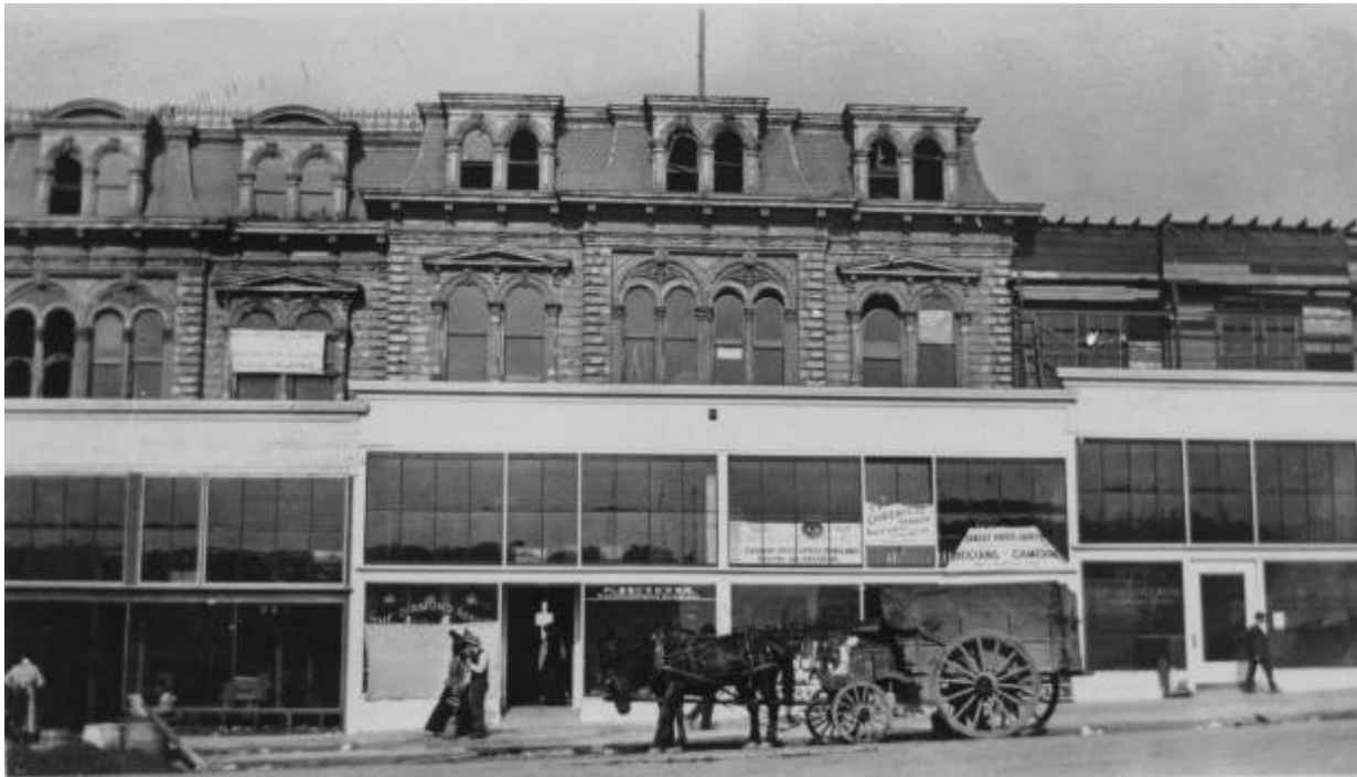
Above: View taken in 1906 of residential flats on Van Ness Avenue with added (post-disaster) ground story commercial spaces. Not extant.
