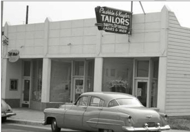
Left: 2621 Judah Street, Facing material at upper story appears to be porcelain enamel or a thin ceramic veneer.
