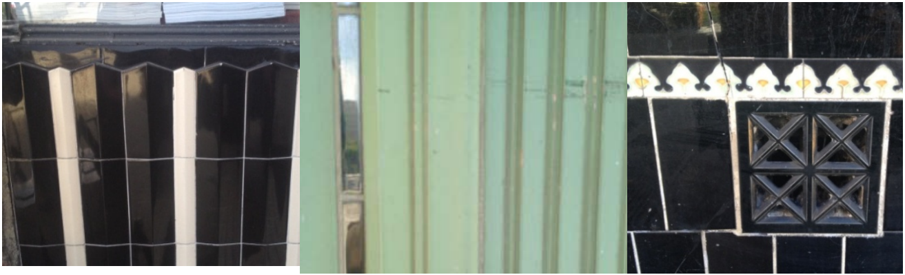
Glazed bulkhead tiles in the 1910s to 1930s were often polychromatic and offered in flush, fluted, and/or embossed forms. Tiles were used widely as a bulkhead material due to their versatility, eye-catching designs, and low initial and maintenance costs.
