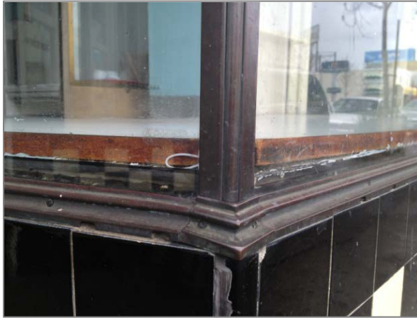
Left: Extruded metal corner bar with mitre cap, San Bruno Avenue.
