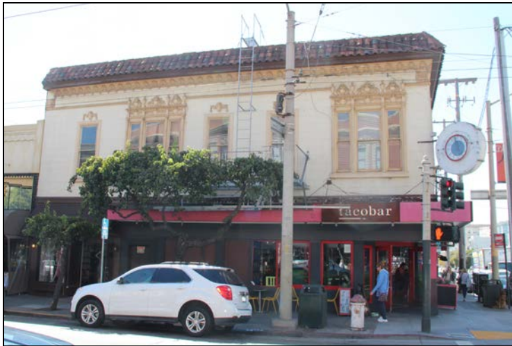
Top: Spanish Colonial Revival, 2401-2417 California displays altered storefronts.
