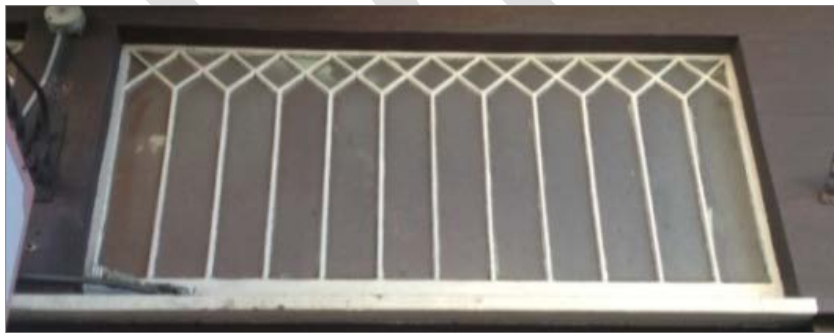
Top row: The transom at 2277 Union Street features arched openings, slender muntins and columned mullions.
