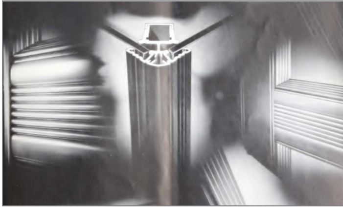
Left: Detail of "Extrudalite" storefront sash frames offered by the L.O.F. glass manufacturers. 1930. Right: Metal storefront sash and transom bars offered by Pittco, 1940. Sources: Glass in Architecture , 1930; Glass and Storefront Products , 1940, Pittsburgh Plate Glass Company.
