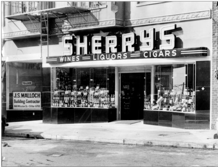
Top left: 254 West Portal Avenue, opened in 1941. It was the chain's 11 th store. The storefront shape is extant, though the Vitrolite cladding was replaced with ceramic tiles in 1970. The neon sign was removed at an unknown date.
