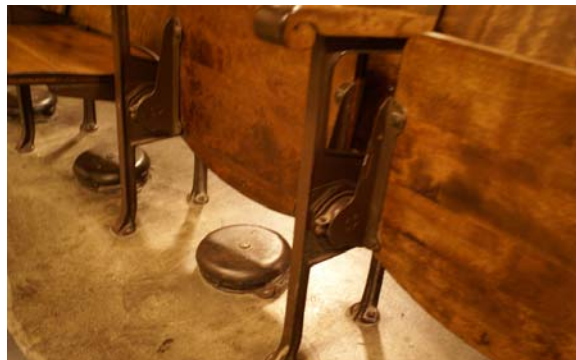
Figure 41. Heating units beneath seats.
