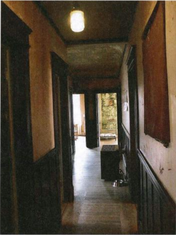
Figure 26 A view down the hallway of Rube Goldberg's apartment shows original finish on the woodwork including wainscoting, surrounds, picture rails, and floor. The hallway, like the rooms off of it, has high cove ceilings. A second gas heater from the third quarter of the 20th Century is set in the hallway.
