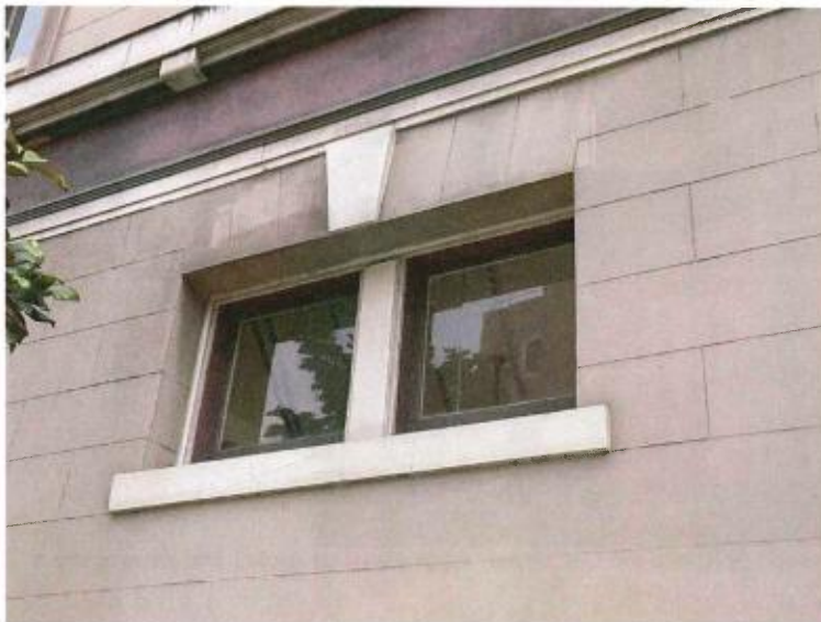
Figure 19 Pair of square raised windows with keystone and incised stucco in imitation of stone set high on the Oak Street elevation's first story.
