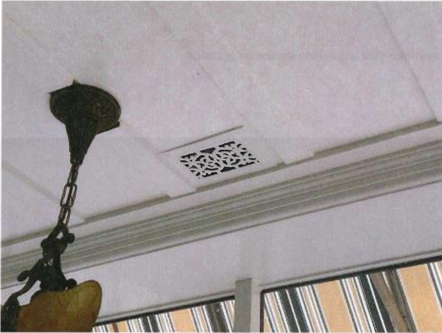
Figure 40 A detail of the wood ceiling moldings and a vent in the front window of 198 Gough Street.
