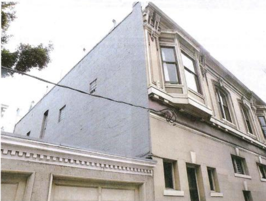
Figure 21 View from Oak Street of the east elevation (left) and the Oak Street, north elevation (right), the garages are a part of the neighboring property.
