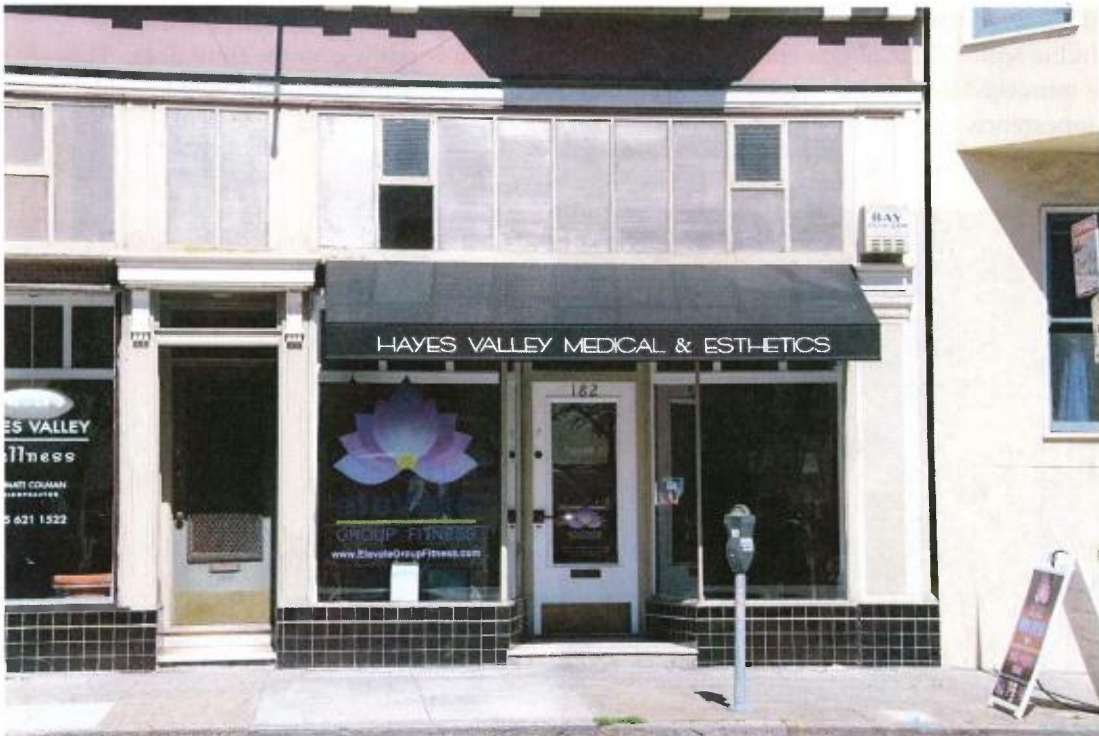
Figure 7 The commercial facade of 182 Gough Street with the residential entrance to 186 Gough St. seen to the north (left).
