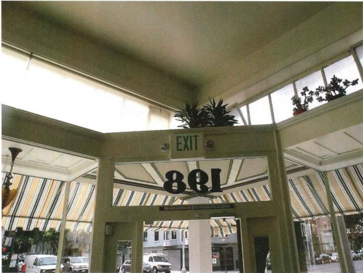
Figure 39 Interior view of the corner commercial space at 198 Gough Street at the corner of Oak Street. Note original finished carpentry on the ceilings of the display area and transom windows of the former saloon. Some doorway framing has been replaced in-kind in a recent rehabilitation by the current tenant.
