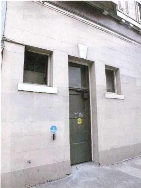
Figure 20 Service door at the east end of the Oak Street elevation. The door is topped by a keystone and flanked by high-set square windows with prominent sills.
