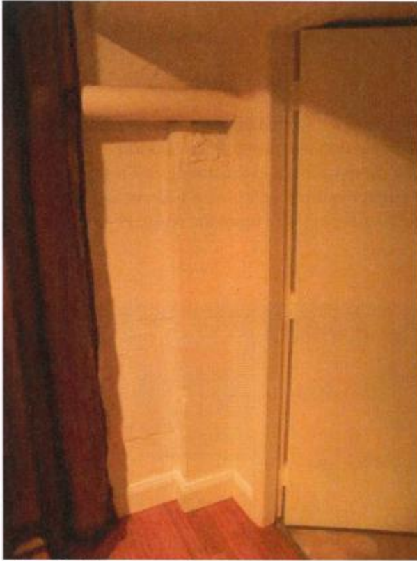
Figure 45 Impressions on the basement wall reveal that the foundations are cast board-formed concrete.
