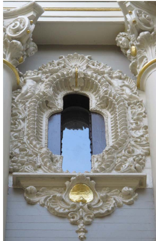
Figure 17: Vertically elongated quatrefoil surround with oval pane (north of bay).
