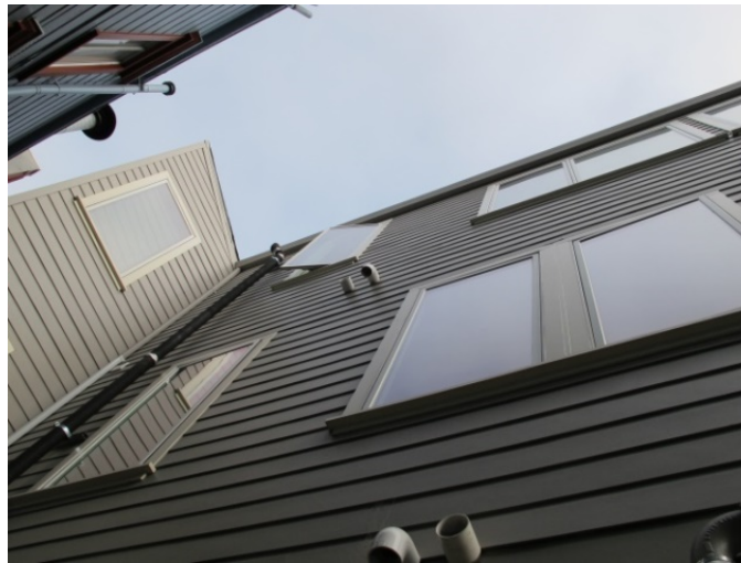
Figure 24: Second and third story fenestration of south façade.
