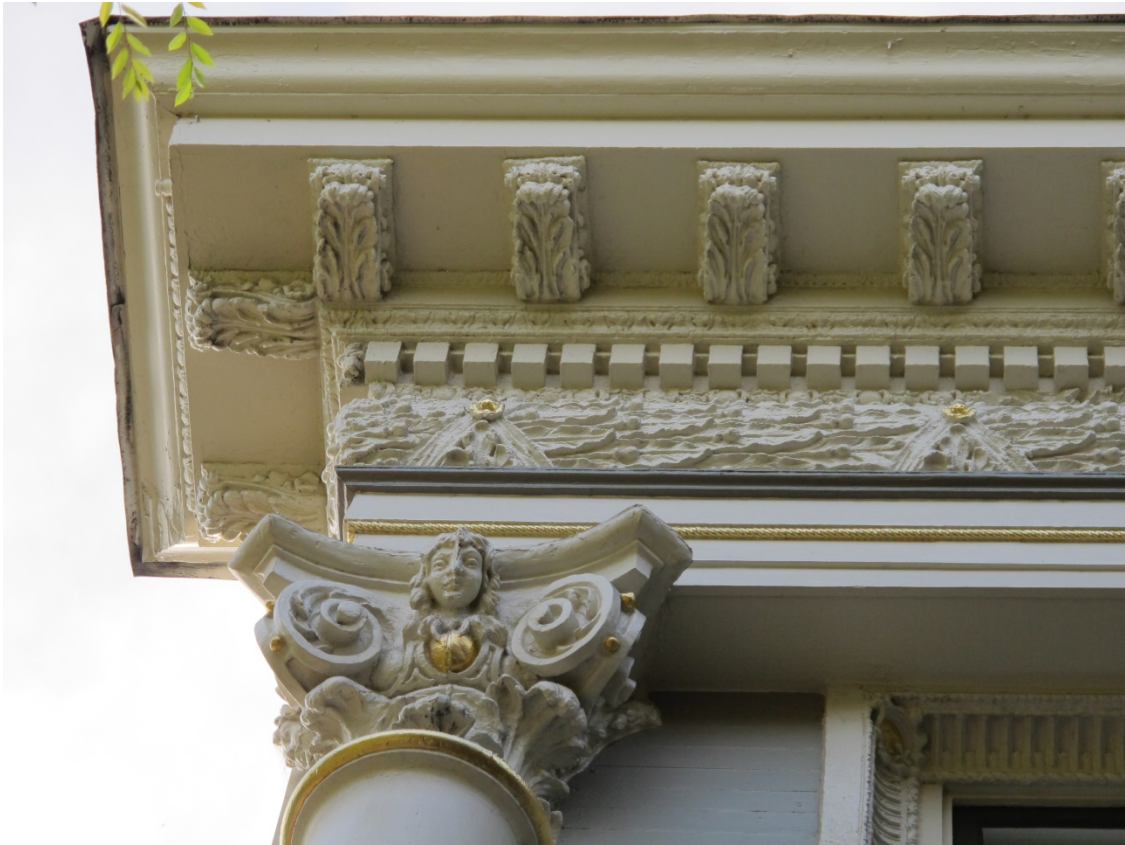
Figure 19: Entablature detail.
