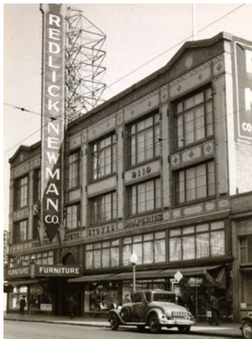
The Redlick-Newman Co. building in 1935. View northeast. San Francisco History Center, San Francisco Public Library (Historical Photograph Collection Photo Id# AAC-7335).
