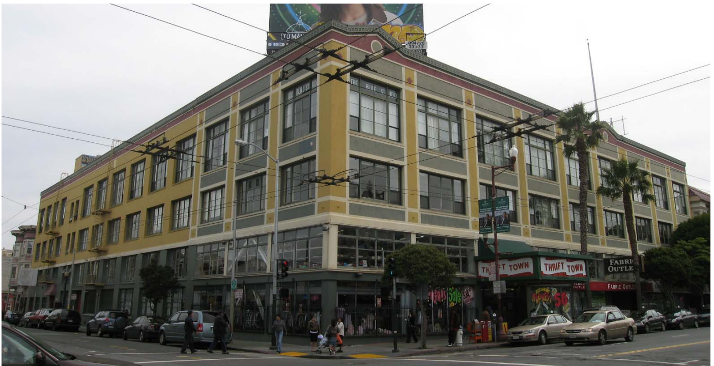
The Redlick-Newman Co. building, located at 2101-2129 Mission Street, in 2011. View southeast. The original structure extended from the corner rooftop pediment to the southern rooftop pediment (located at right), and from the corner east to the break in the larger windows (located at left). Additions to the original building include the southernmost section (located at far right) and the easternmost section (located at far left). San Francisco Planning Department.
