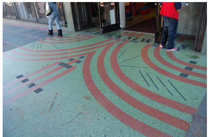
The customized terrazzo floor paving at the main entrance of the Redlick-Newman Co. building. View northeast. San Francisco Planning Department.
