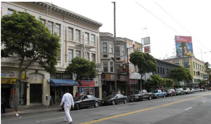
The east side of Mission Street. View southeast towards 17 th Street. The concrete apartment building located at the left was constructed in 1914. San Francisco Planning Department.
