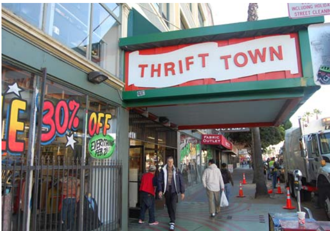
The box marquee and ground-floor plate-glass display windows of the Redlick-Newman Co. building. View south. San Francisco Planning Department.
