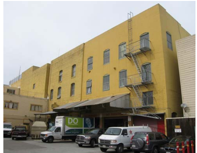
The south-facing side of the building at the interior of the block. View northeast from Capp Street. The building's three sections include: the store with Mission Street frontage at left; the original warehouse at center; and the rear addition at right. San Francisco Planning Department.
