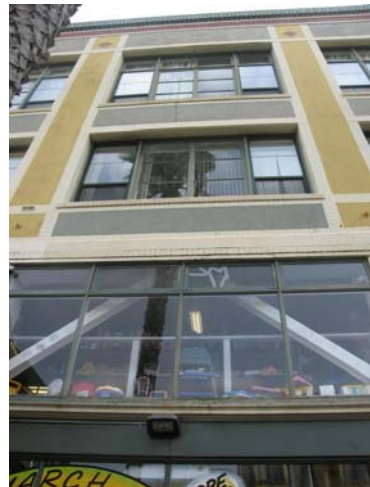
Bands of large divided metal-sash windows with brick water tables, located at the Mission Street façade of the Redlick-Newman Co. building. View northeast. San Francisco Planning Department.
