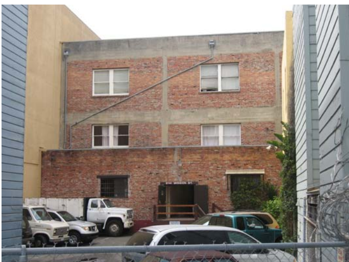
The back of the Klopstock Bros. furniture store. View west from Capp Street. The ell-shaped warehouse abuts to the left. San Francisco Planning Department.
