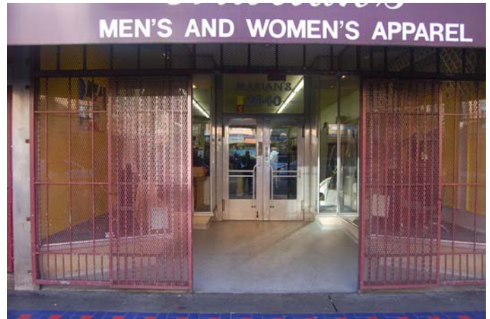
The building with a “Visual Front” located at 2040-2042 Mission Street. Views west. Materials and features include: structural glass facing; steel trim, rectangular metal windows; deep angled vestibule; plate-glass in metal frames; overhanging window displays; metal sash doors. San Francisco Planning Department.
