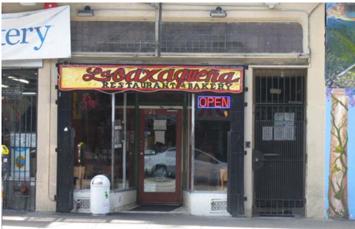
Typical storefront, located at 2128 Mission Street (built 1913). Includes: plate-glass windows in custom metal frames with fretted inlays that match the façade; decorative grills at bulkhead vents; an angled vestibule and wood sash door; and a decorative multi-light clerestory, which runs the width of the building above the first story. San Francisco Planning Department.
