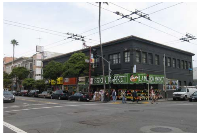
The northeast corner of Mission and 17 th Streets. View northeast. The corner commercial building was constructed or expanded in 1922. San Francisco Planning Department.
