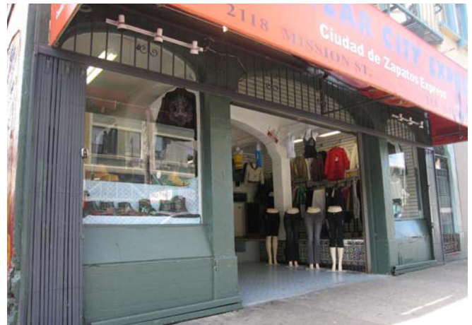
Customized storefront for a "bazaar", located at 2118 Mission Street (built 1912). Includes: an arched entrance and arched plate-glass windows; bulkheads clad in decorative floral tile (painted over at street face); and a deep arcade entrance with decorative floral floor tile. Consistent with the building's overall Mission Revival styling. San Francisco Planning Department.
