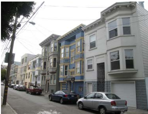
Residential buildings located on the west side of Linda (formerly Angelica) Street, south of 19 th Street. View southwest. San Francisco Planning Department. DPR 523L (1/95)
