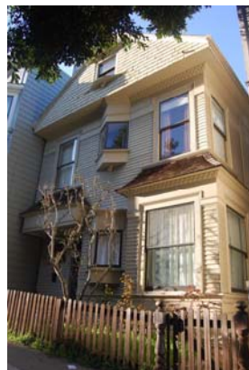
Shingle-style house located at 3746 20 th Street. View north. San Francisco Planning Department.
