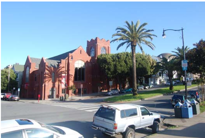
Mission Park Congregationalist Church located at the southeast corner of Dolores Street and 19 th Street. View southeast. San Francisco Planning Department.
