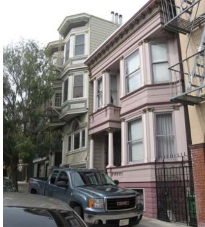
Residential buildings located on the north side of 20 th Street, between Dolores Street and Guerrero Street. View northwest. San Francisco Planning Department.
