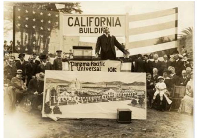
Mayor Rolph speaking in 1914, at the groundbreaking for the California Building of the Panama Pacific International Exposition. San Francisco History Center, San Francisco Public Library (Historical Photograph Collection Photo Id# AAD-7317).
