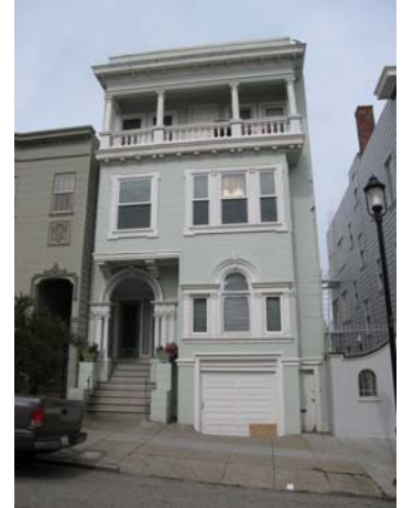
Residential building located on the north side of 20 th Street, west of Guerrero Street. View north. San Francisco Planning Department.
