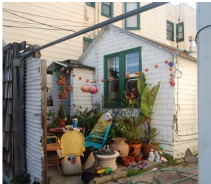
Refugee-style cottage located at 146 Linda (formerly Angelica) Street. View west. San Francisco Planning Department.
