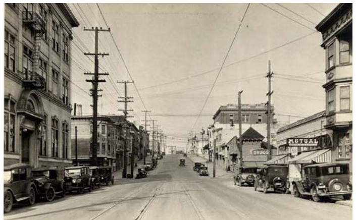
Guerrero Street in 1928. View north towards 14 th Street. All of the buildings that appear in the photograph were constructed to replace properties destroyed in the 1906 fires. San Francisco History Center, San Francisco Public Library (Historical Photograph Collection Photo Id# AAB-3941).
