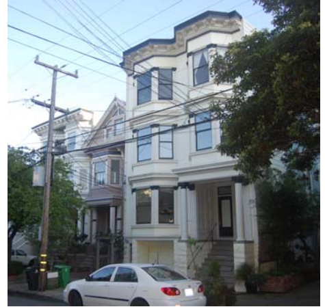
Residential buildings located on the south side of Cumberland Street. View southeast. San Francisco Planning Department.
