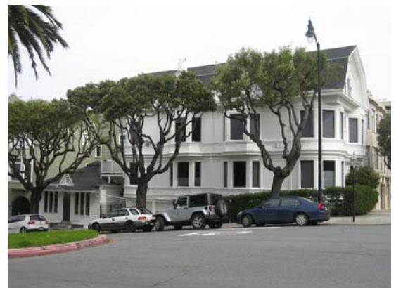
Dutch Colonial/Colonial Revival-style residential flats located at 96-98 Cumberland Street and the backyard cottage located at 635 Dolores Street. View east. San Francisco Planning Department.
