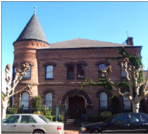
Landmark #58: SF Gas & Light Co., 3640 Buchanan St.
