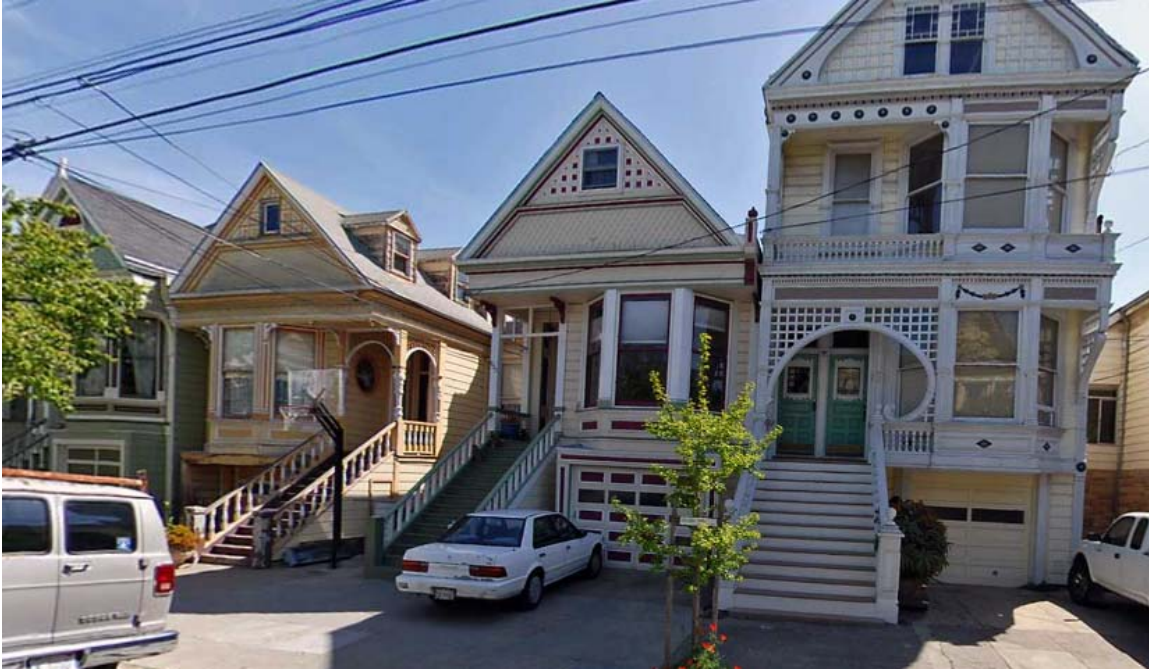
West side of York Street between 21 st and 22 nd Streets.
