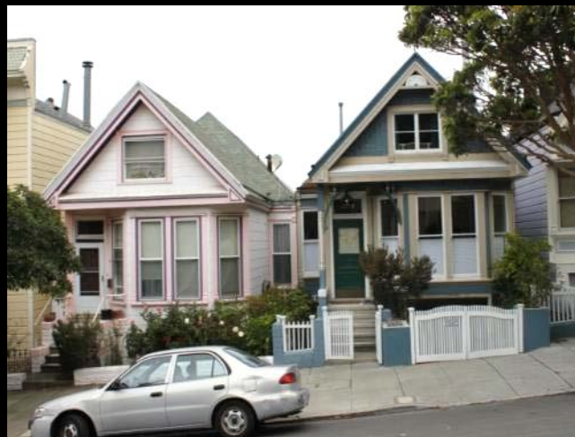
554 and 558 Liberty Street (built 1897)
