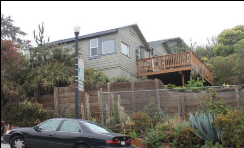
Earthquake shack dwelling at 300 Cumberland Street
