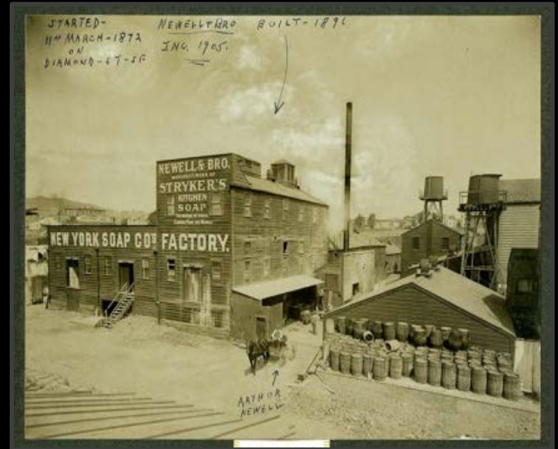
New York Soap Company works on Diamond Street, ca. 1890. (Date written on photo inaccurate.)
