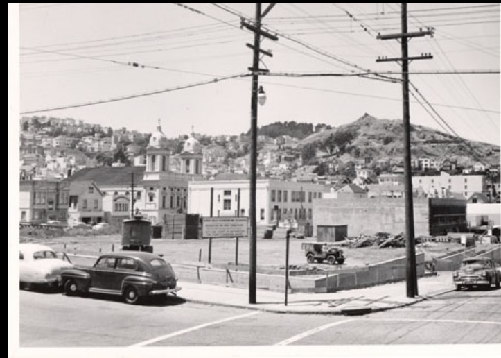
Eureka Valley playground and recreation center under construction, ca. 1954.
