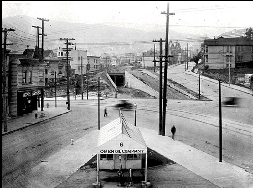
Twin Peaks Tunnel nearing completion, ca. 1917
