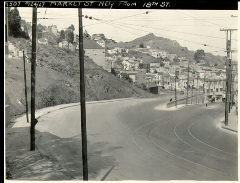
Market Street extension looking northeast from 18 th Street, 1927
