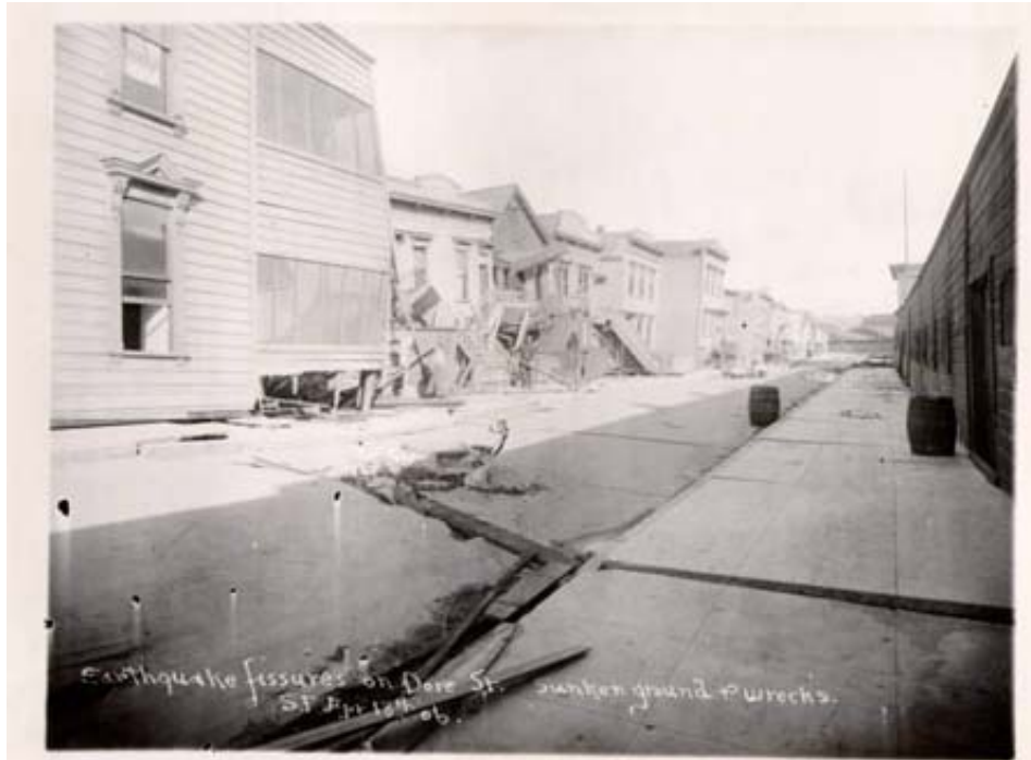
Figure 11. Earthquake fissures and collapsed wood-frame buildings on Dore Street, 18 April 1906. (Source: San Francisco Historic Photograph Collection, SFPL, AAC-3170)
