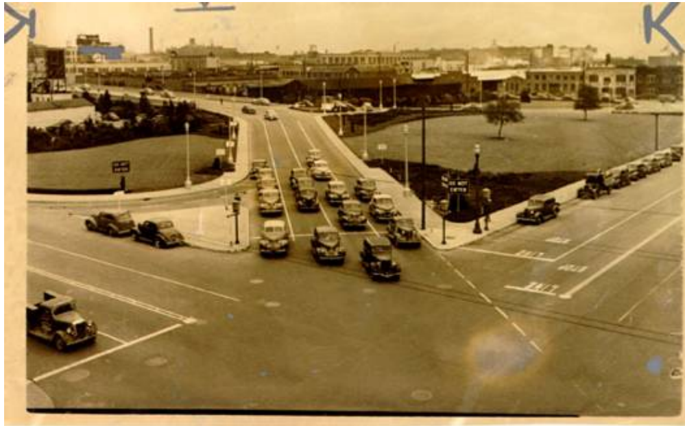
Figure 25. Approach to the San Francisco-Oakland Bay Bridge at Harrison and 5 th streets, 8 December 1942.
