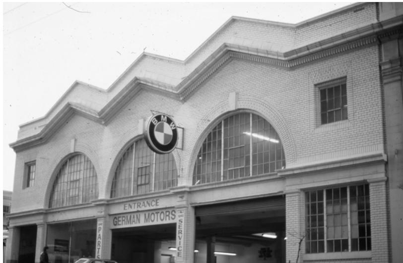
St. Francis Garage, 1240 Post Street, built in 1916 to designs by Sylvain Schnaittacher. Photo by William Kostura, 1983. This was a Class A steel-frame building with a brick front. It had the usual three-bay composition and industrial steel sash windows, but its zig-zag parapet and cornice were unique. This building and the adjacent Heald's College, also by Schnaittacher, were demolished in 1983.
