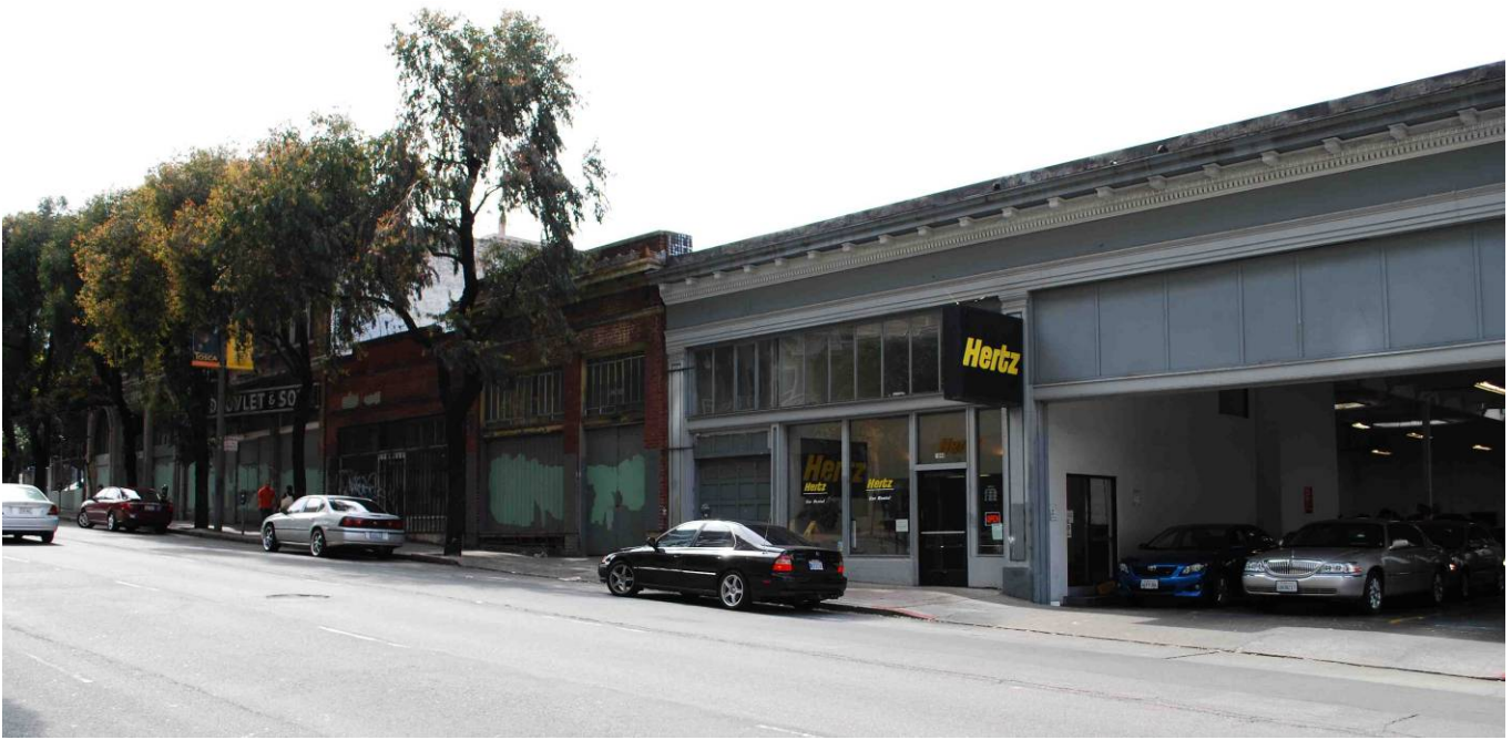
View of 1644-1670 Pine Street, looking northwest. #1644 is at far right.
