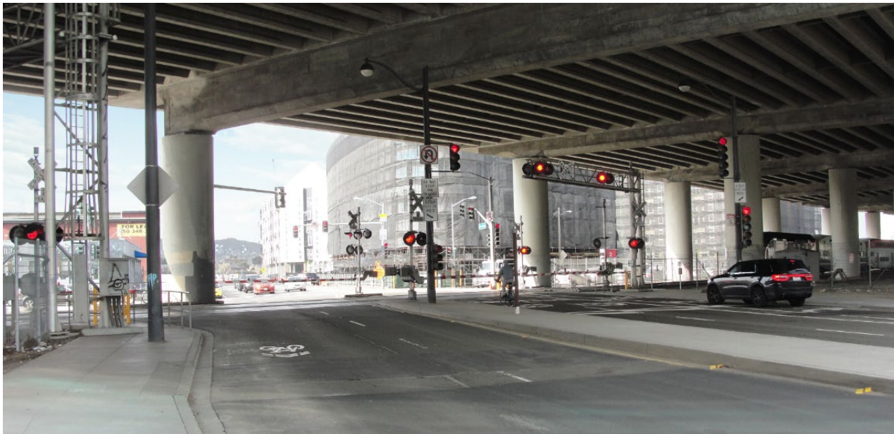
Figure 1: 16 th Street At-Grade Rail Crossing
