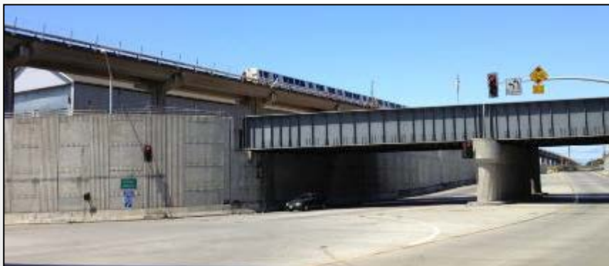
Existing Grade-Separation Near West Oakland Bart Station at 7 th Street
