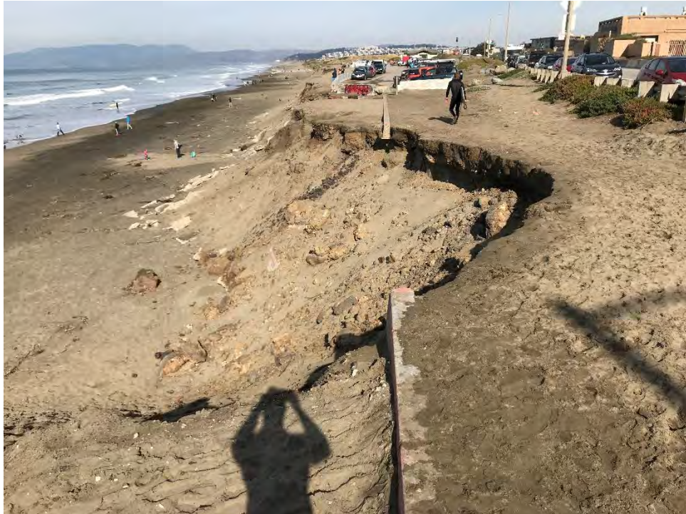
North Parking Lot, erosion and rubble north of Sandbags
