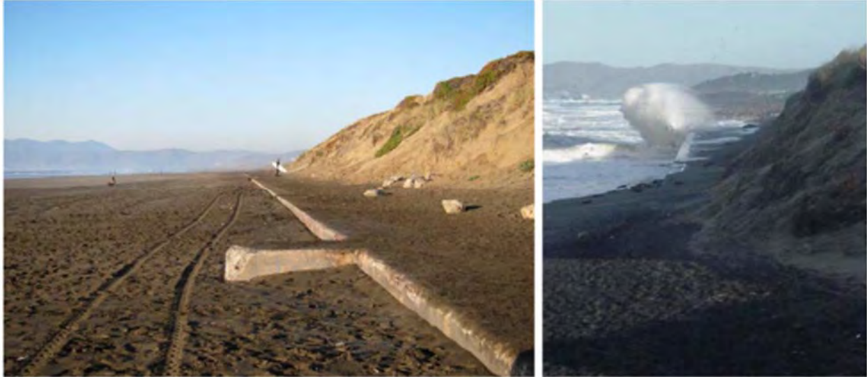
Figure 4 Taraval seawall in fall 2011 (left, © E. Vandebroek) and winter 1998 (right, © B. Battalio)
