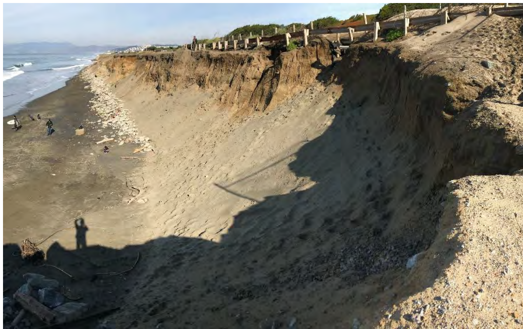
Erosion and rubble north of 2010 Emergency Bluff Toe Protection
