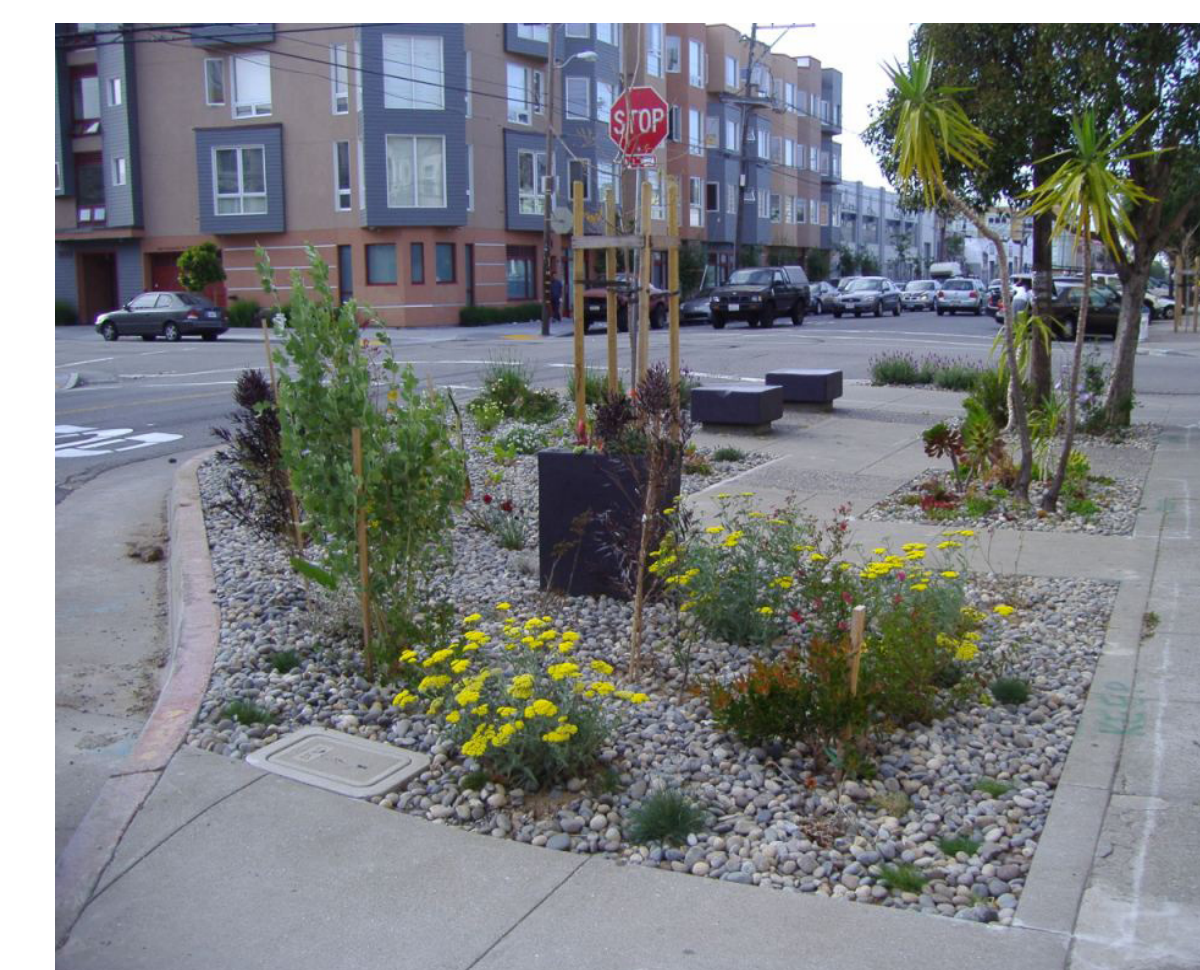
STORMWATER PLANTERS & LANDSCAPING
