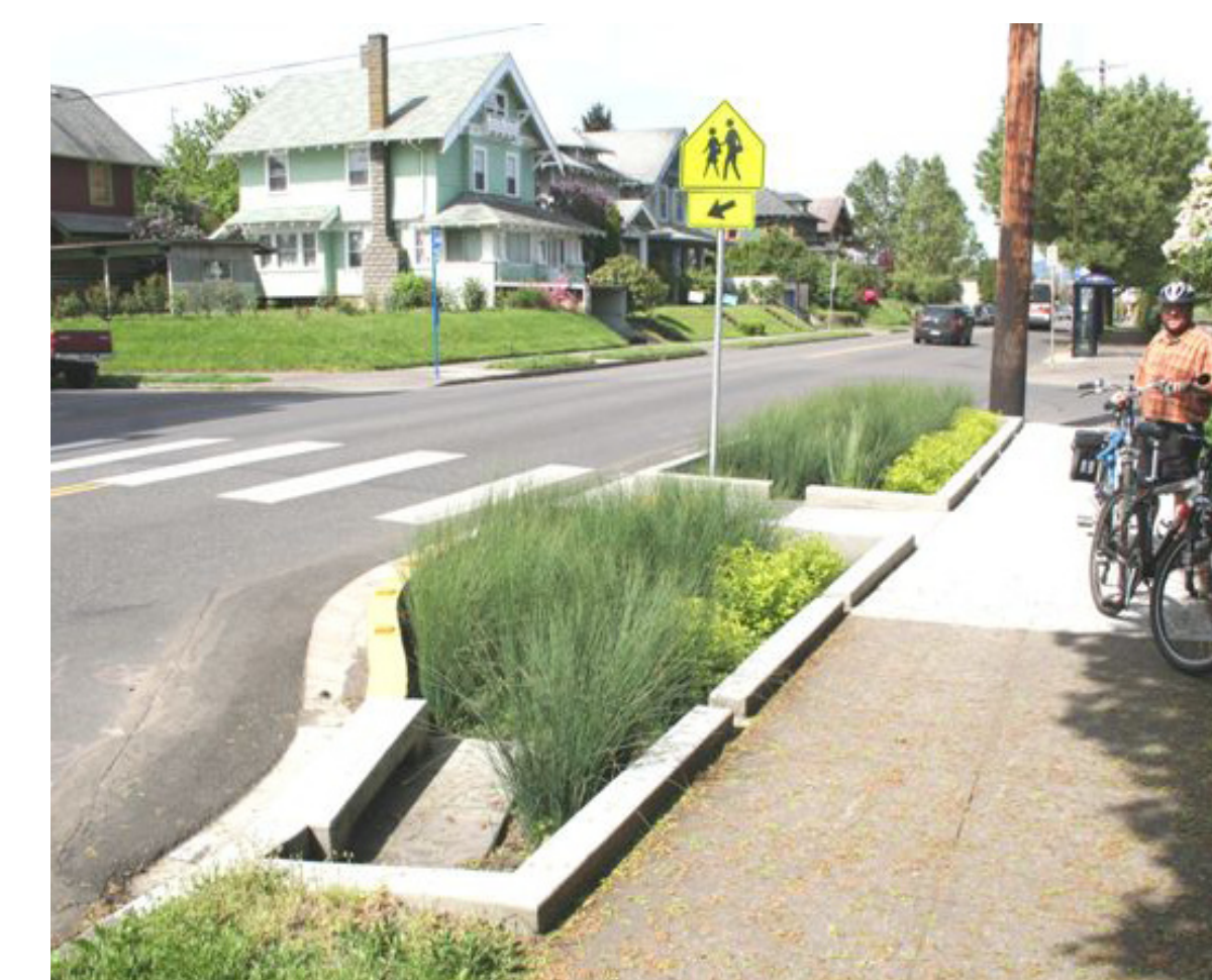
STORMWATER PLANTERS & CURB EXTENSION
