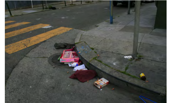
11 Lack of cleanliness and maintenance is found at some locations.
