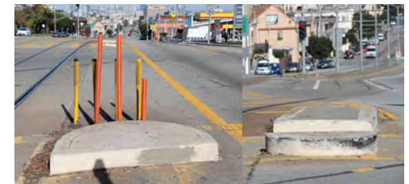
Pedestrian refuges too narrow, unprotected, and poorly marked.
