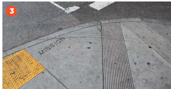
Vehicles often run over the curb when making a right turn, endangering pedestrians.
