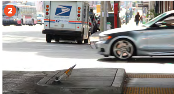
Ineffective marking of pedestrian refuge. No real protection from high-speed vehicles.
