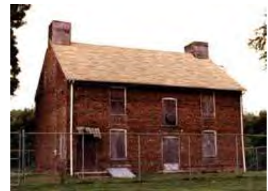
A view showing the exterior of the Brearley House, New Jersey, in its mothballed condition. Photo: Michael Mills, Ford Farewell Mills Gatsch, Architects.
