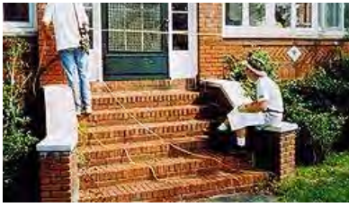
Documenting a building's history and assessing its condition provide information to set priorities for stabilization and repair, prior to mothballing. Photo: NPS files.
