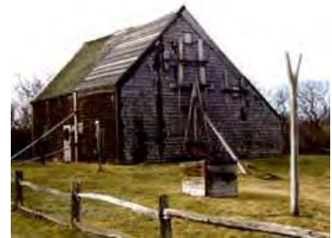
Buildings seriously damaged by storms or deterioration may need to be braced before architectural evaluations can be made. Photo: John Milner Architects. Photo: NPS files
