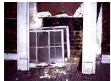
Loose or detached elements should be identified, tagged and stored, preferably on site. Photo: NPS files
