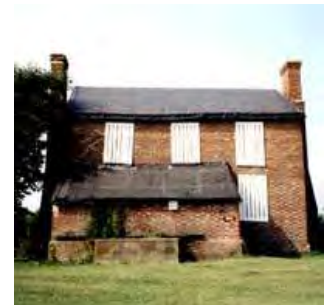
Appropriately mothballed historic building. Photo: NPS files.
