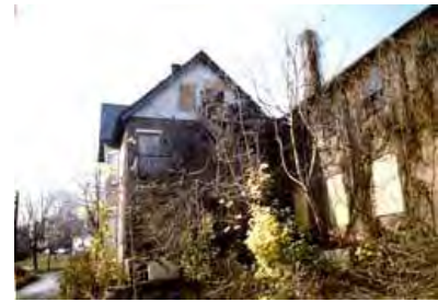
Boarding up without adequate ventilation and maintenance has accelerated deterioration of this property. Photo: NPS files.
