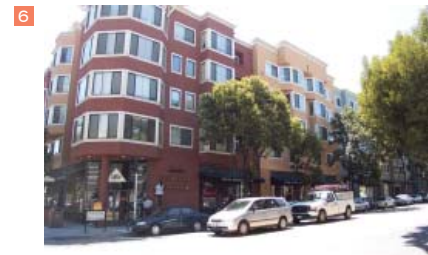
Although constructed on a large lot, this building façade replicates the traditional 25 - 50 foot-wide lot pattern through changes to the plane, color and roof line.
