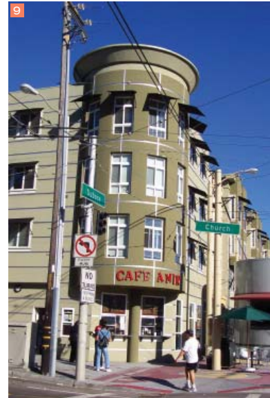
Corner Tall tower / bay element establishes a visual landmark at an important street intersection
