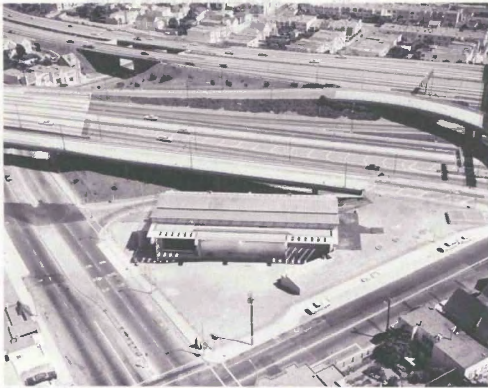
Aerial view of the Glen Park BART station, 1970. Courtesy of San Francisco Public Library.
