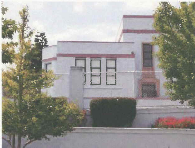
View west toward the school's east elevation, 2009.
