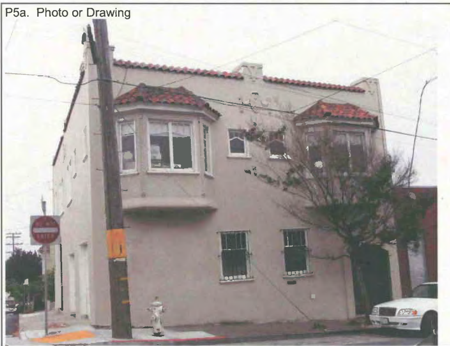
P5b. Description of Photo: View of the façade and the east elevation from Chenery Street; June 2, 2009.
