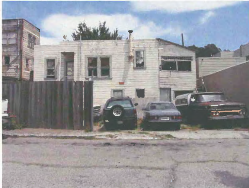
View north on Kern Street toward 23 Brompton Avenue, 2009.
