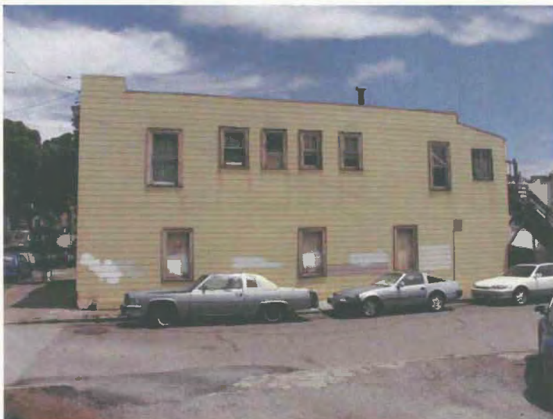
View north on Kern Street toward 25 Brompton Avenue, 2009.
