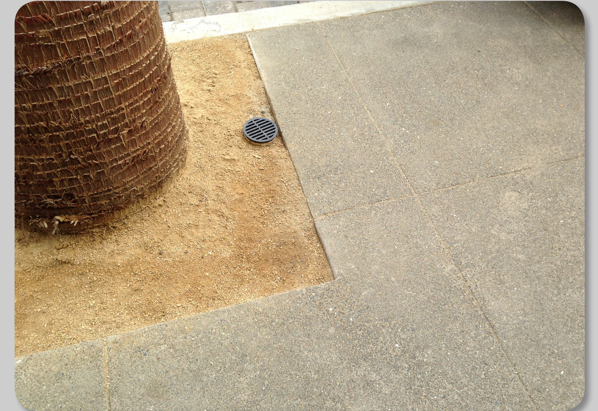
NEW CONCRETE SIDEWALKS
