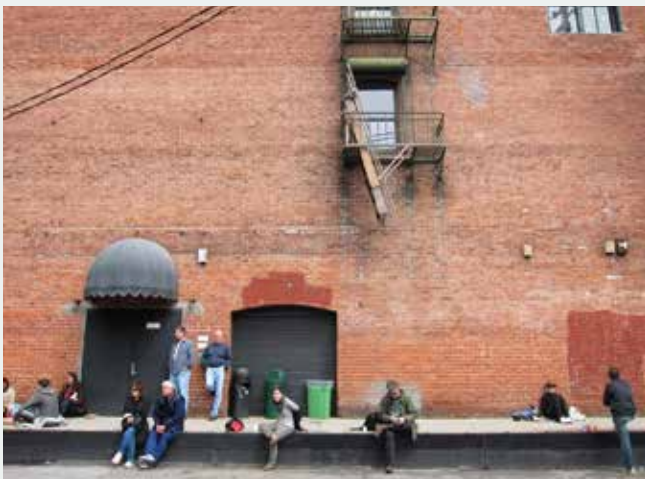
Loading dock near Little Skillet. Photo credit: Kendra Aronson.
