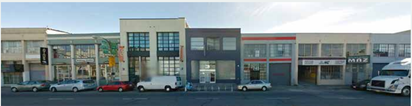
Bryant Street elevation. Photo by Google Maps
