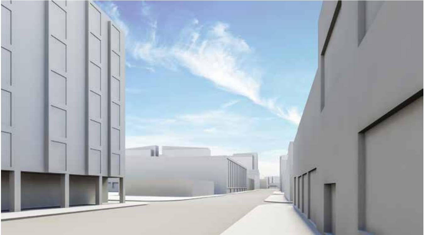
C.1 View from Fourth and Bryant looking southeast (existing).
